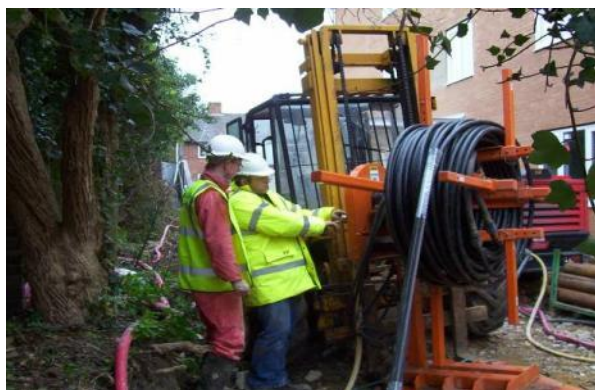
Fig 3 Installing ground loops
