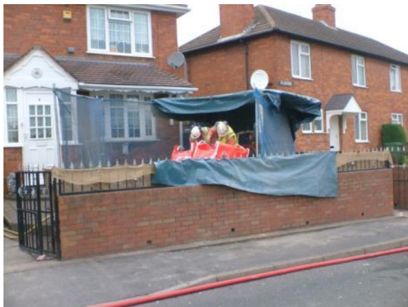
Fig 2 Drilling to stabilise mineshaft in back garden
