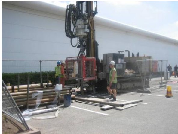
Fig 1 Sonic drilling on former open cast mine
