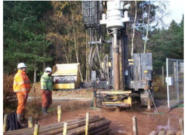
Fig 3 Large diameter well installation
