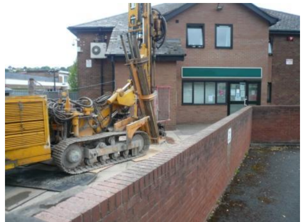
Fig 4 Drilling to install ground loops
