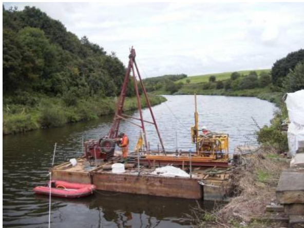
Fig 2 Drilling for site investigation at Northwich
