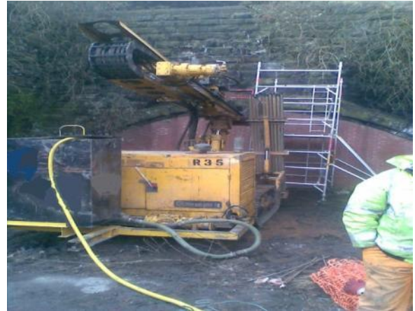
Fig 3 Drilling for Tunnel Infill
