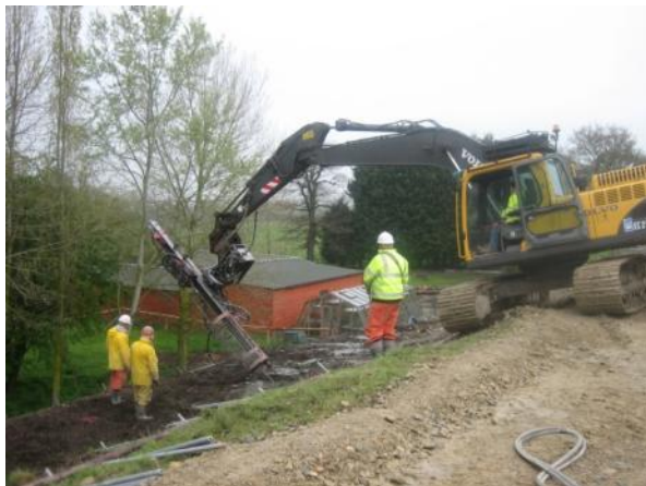
Fig 2 Installing soil nails
