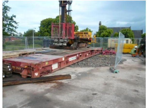
Fig 3 Drilling to a stabilise mineshaft, Telford
