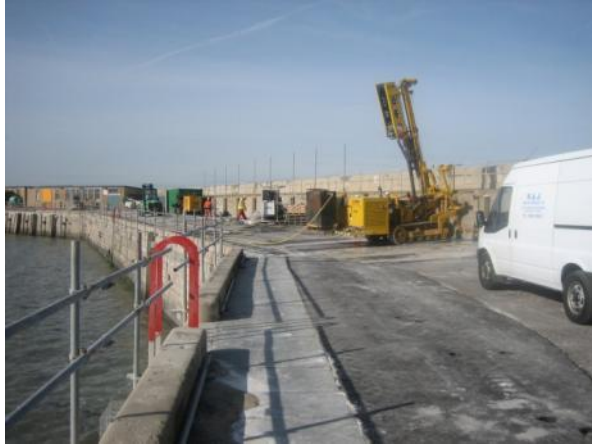
Fig 1 Drilling to stabilise harbour arm wall
