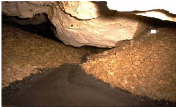
Fig 2 Gravel barrier installation
