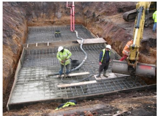
Fig 4 Reinforced Concrete Cap Construction
