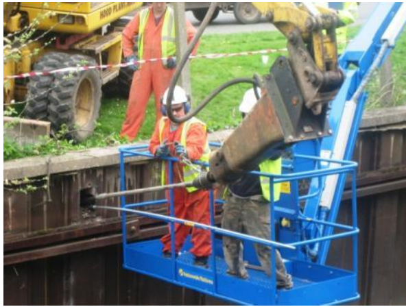
Fig 1 Installing Platipus Anchors for sheet piles
