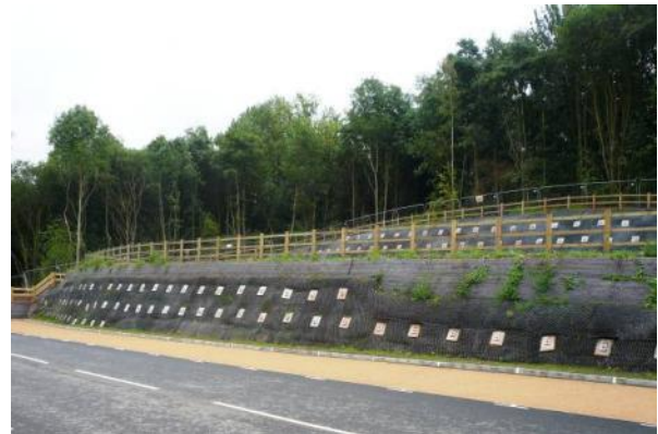
Fig 4 Finalised soil nail wall
